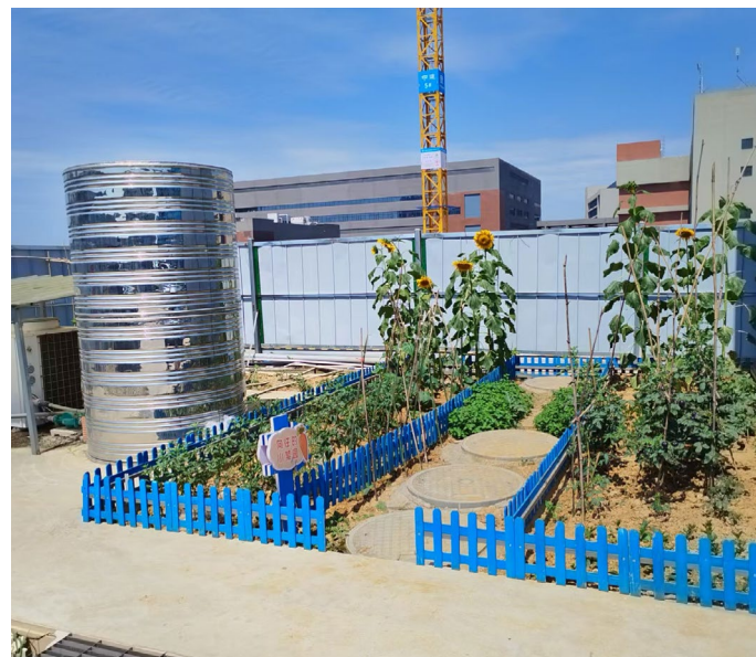
Prefabricated Septic Tank and Air-Source Water Heater
